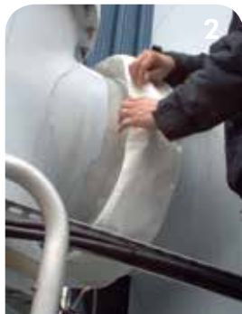
Leak sealing with soft cover application and valve
